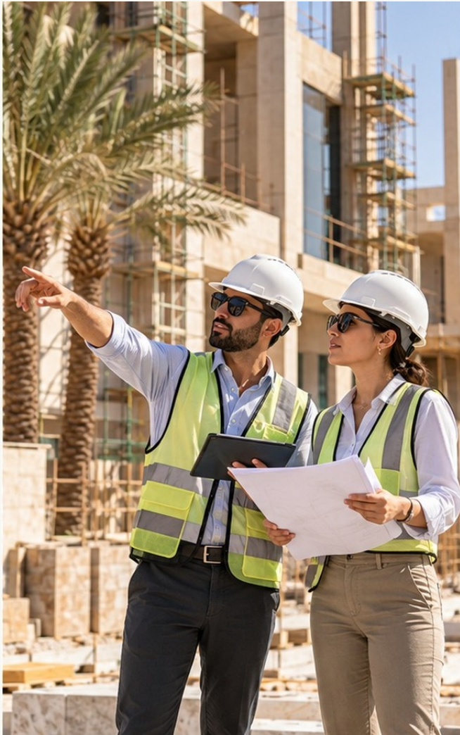
Site progress and execution
